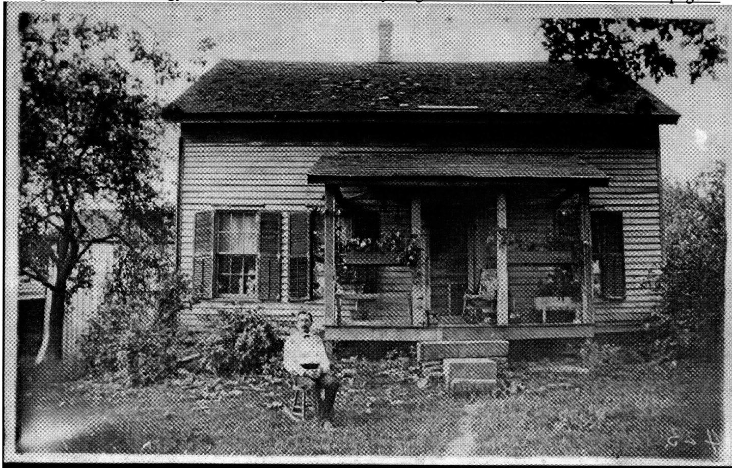
Drakesburg: Cliff Moore House --no date
